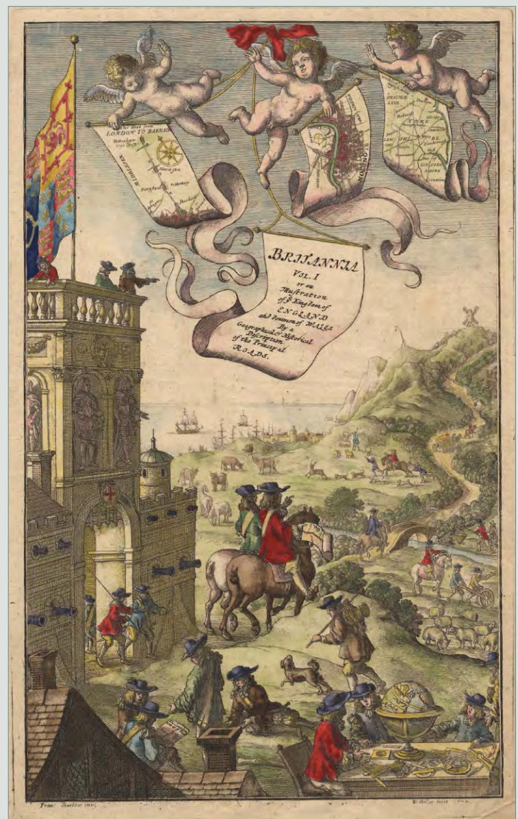
Figure 4. Frontispiece of John Ogilby's Britannia (London, 1675). Amidst the bustle of this English scene, a master surveyor (on horseback) instructs two others (on foot) as they push the perambulator or measuring wheel—Ogilby's "Wheel Dimensurator"—to ascertain the length of a crossroad (lower right). Above all, three putti with banners advertise the atlas and its maps. Although Ogilby's name is nowhere to be found, two names do appear on the bottom: Francis Barlow, who drew the frontispiece ("Fran. Barlow inv."); and Wenceslaus Hollar (1607–1677), one of London's leading engravers, who engraved it ("W. Hollar fecit 1675").
